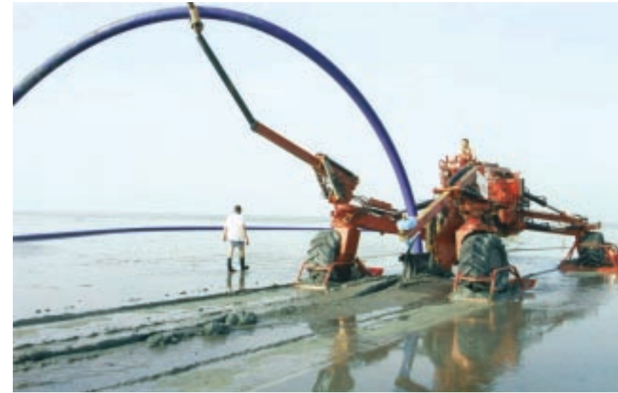
The Foeckersperger cable plow installing the pipe through the mud flats.
