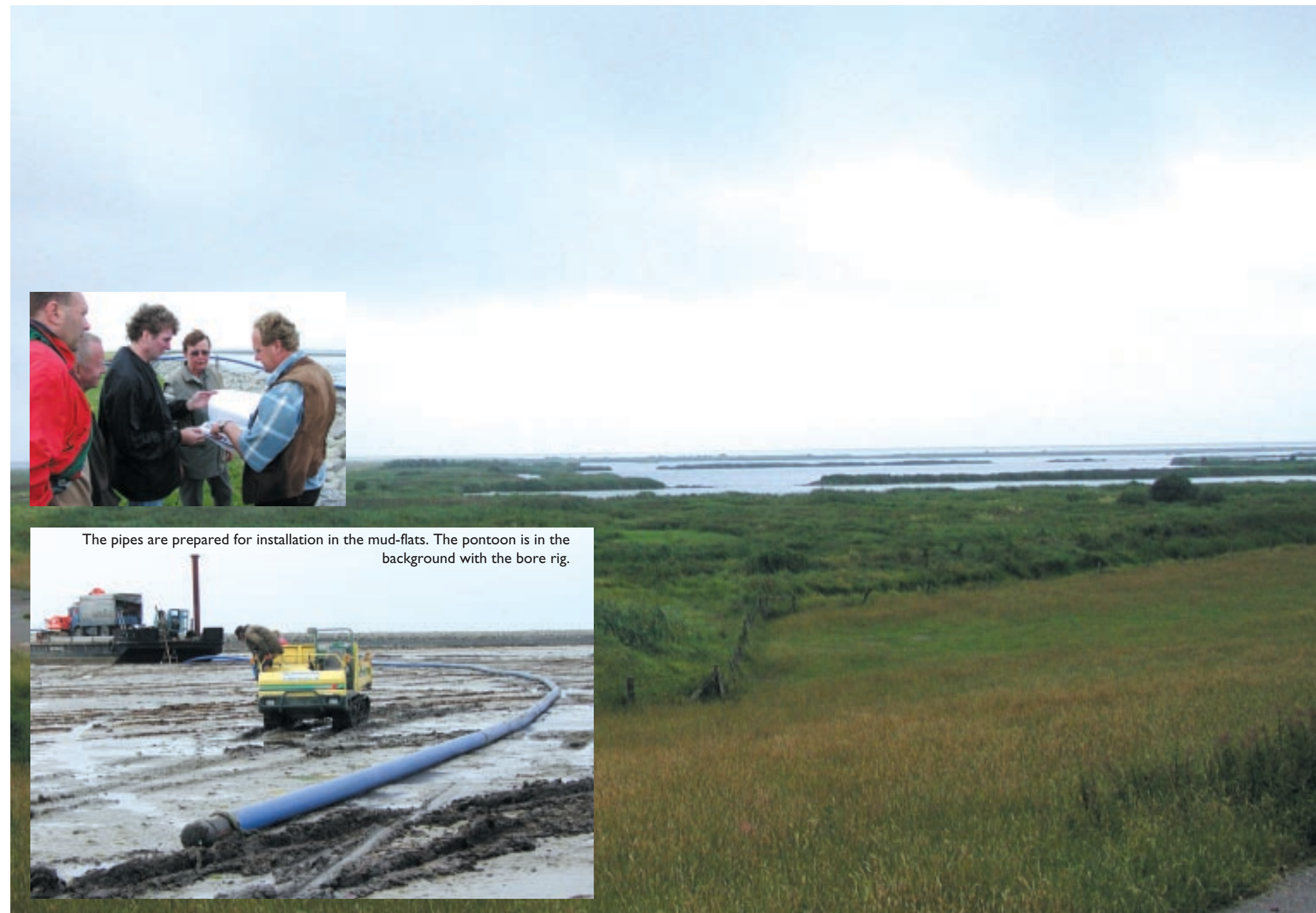
The Foeckersperger cable plow installing the pipe through the mud flats.
