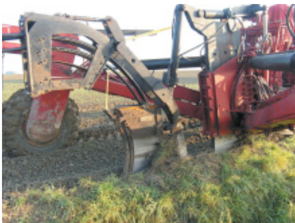
Plowing in of the cables
